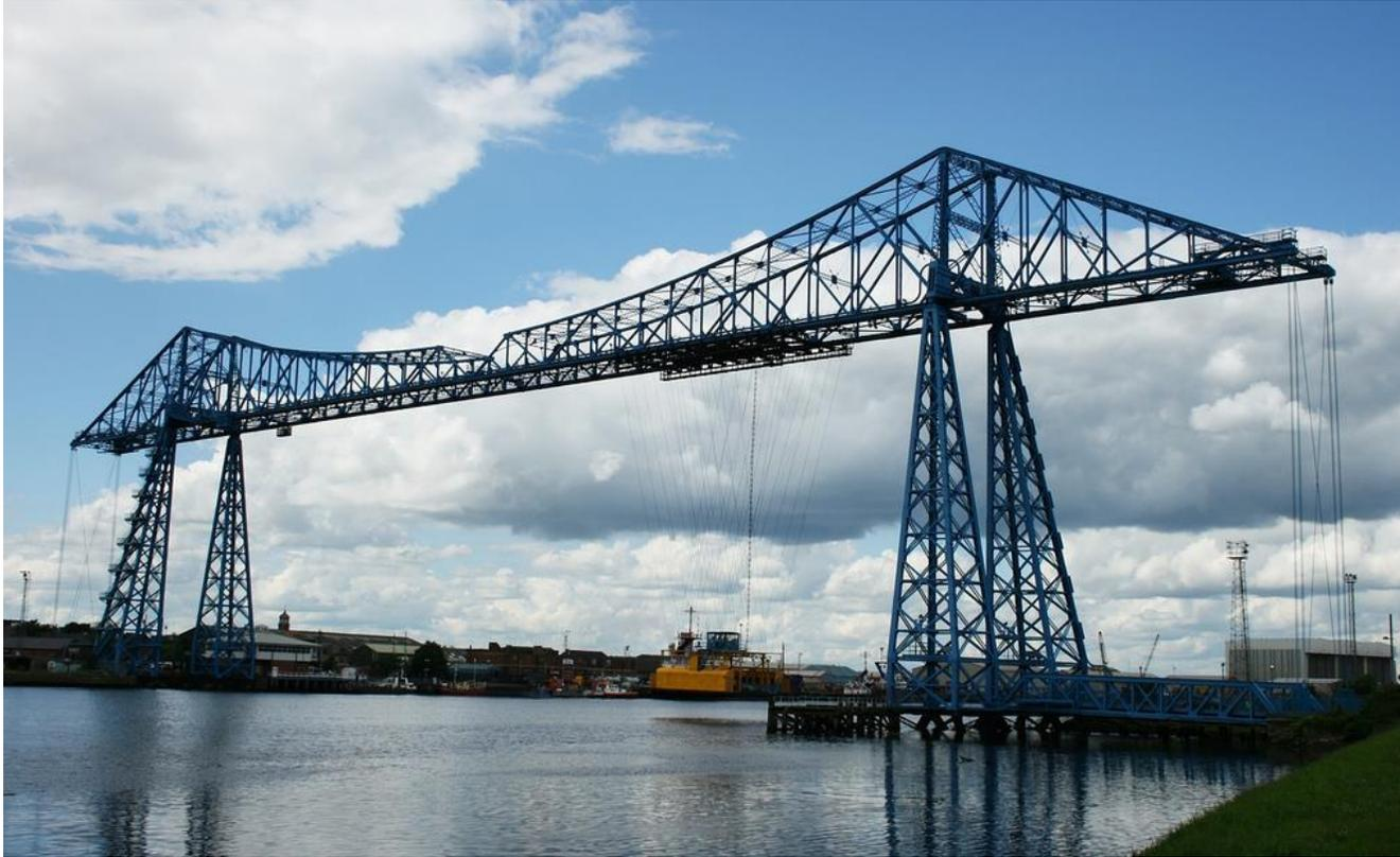
The Transporter Bridge is a special type of bridge that carries a travelling car or gondola, suspended from the bridge across the river in less than 90 seconds. It is more than 100 years old! Have you ever been on the Transporter bridge?
