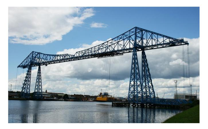
The Transporter Bridge is a special type of bridge that carries a travelling car or gondola, suspended from the bridge across the river in less than 90 seconds. It is more than 100 years old! Have you ever been on the Transporter bridge?
